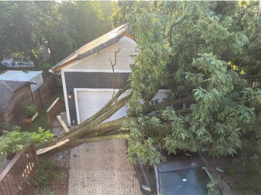
Tree down in St. Charles in July. There were A LOT of trees down and cosmetic damage during the February and July tornados.
