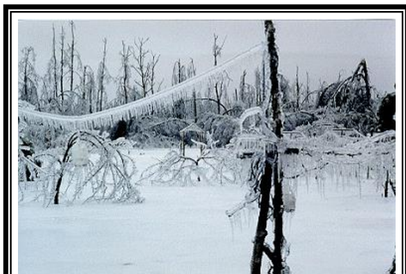
Above ground lines are especially susceptible to damage by ice storms. The loss of power has a ripple affect to many other properties. Source: Matthew Masek, University of Nebraska
